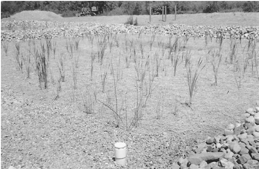
Figure 16.6 On-site subsurface flow constructed wetlands recently planted at Ten Stones near Burlington, Vt.
