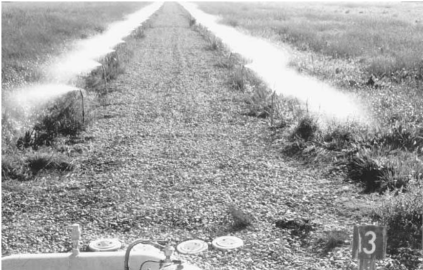
Figure 11.3 Spray heads for distribution of wastewater onto overland flow slopes at city of Davis, Calif.
