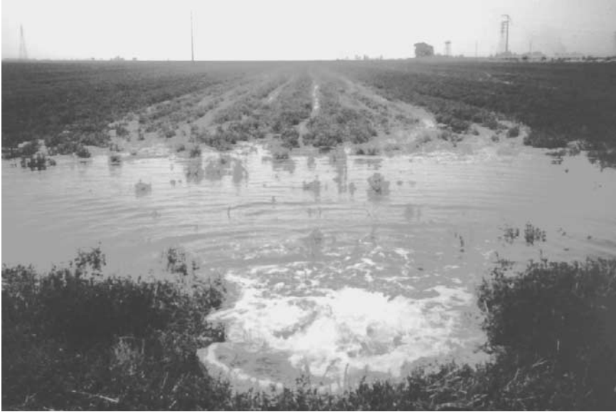
Figure 9.6 Typical discharge valve for border strip application.
