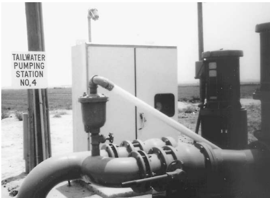
Figure 9.3 Typical tailwater pumping station.
