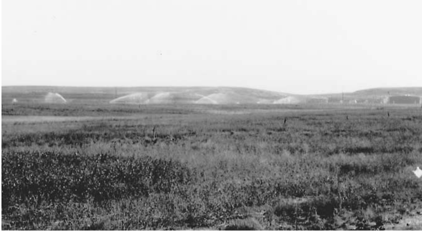
Figure 13.2 Solid set sprinklers apply tomato-processing wastewater to overland flow slopes.
